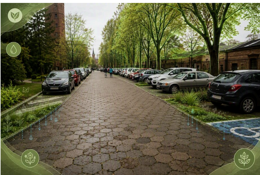
Road with authorised car traffic and designated parking spaces (Source: U-Mob Project, 2018)
